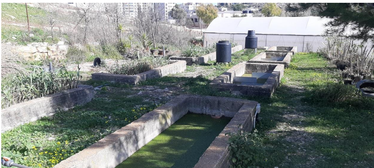
Figure 6: Pilot system of vfcWs and dWSPs at Birzeit University campus
